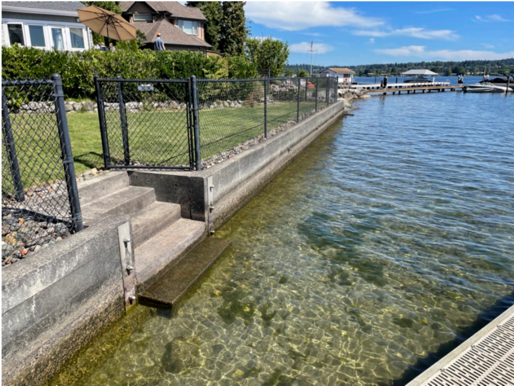
Photo 3 - Existing shoreline conditions looking north.
