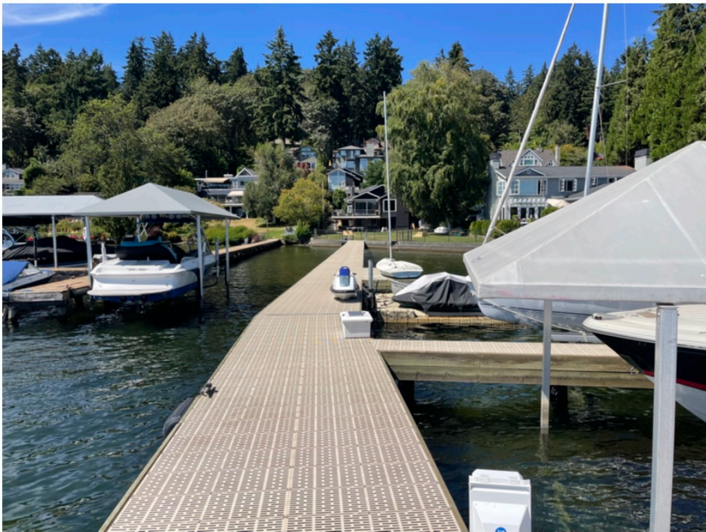
Photo 2 - Existing dock looking landward.
